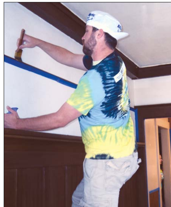
Jake Eddy, Clark Construction
